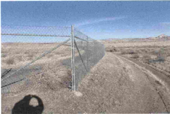
Perimeter of the fence looking North from East at entrance gate
