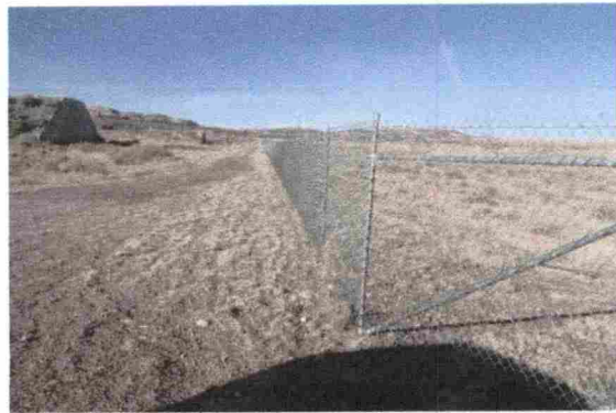
Perimeter of the fence looking West from East Entrance Gate
