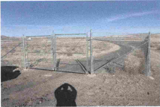
East Entrance Gate looking West
